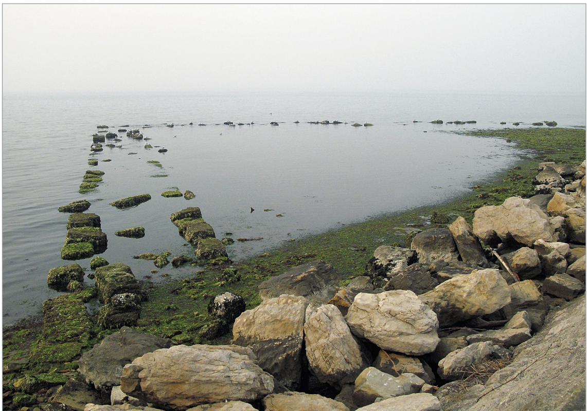
Fig. 14. Roman port structure at Viližan, 23 Feb 2008, 16.00 hours, 65 cm below mean sea-level (photograph: Andrej Gaspari).
